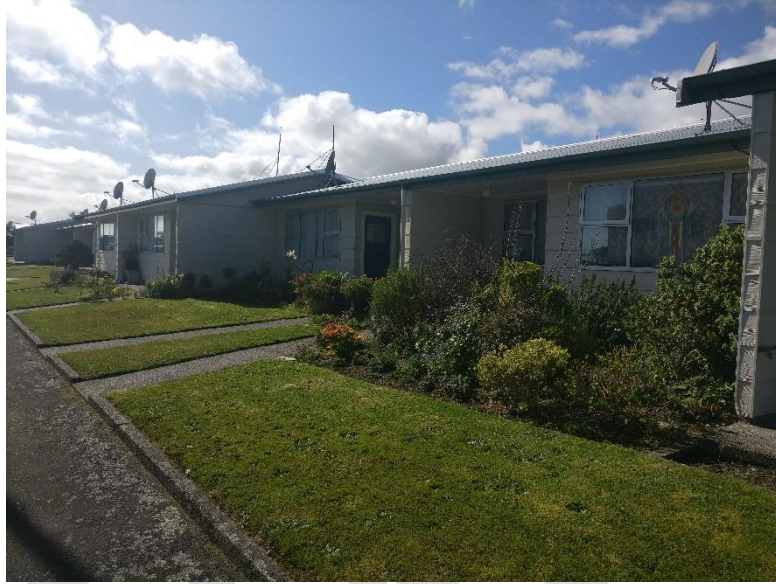
Units at Sewell Street
