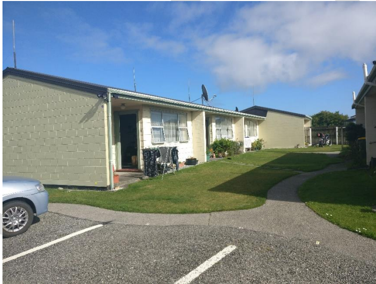
Units at Tancred Street
